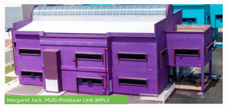
Like its sister building, the Margaret Jack MPU was configured as a twin to the Caroline Sophia Cowie MPU. This unit also comprises two (2) levels with four (4) business units on each floor, ranging from 53.2 m<sup>2</sup> (573 ft<sup>2</sup>) to 130.1 m<sup>2</sup> (1,400 ft<sup>2</sup>). All common services and supporting infrastructure are the same as the Caroline Sophia Cowie MPU.
