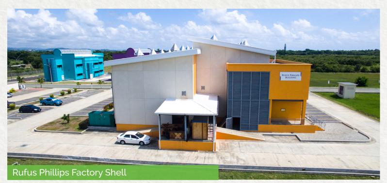
Built as a twin to the Isaac T. Mc Leod Factory Shell, the Rufus Phillips Building is also ideal for light manufacturing and consists of 278.71 m<sup>2</sup> (3,000 ft<sup>2</sup>) of factory space and 111.5 m<sup>2</sup> (1200 ft<sup>2</sup>) of office space. It has been constructed with all common services, welfare and safety facilities, utilities and amenities.
