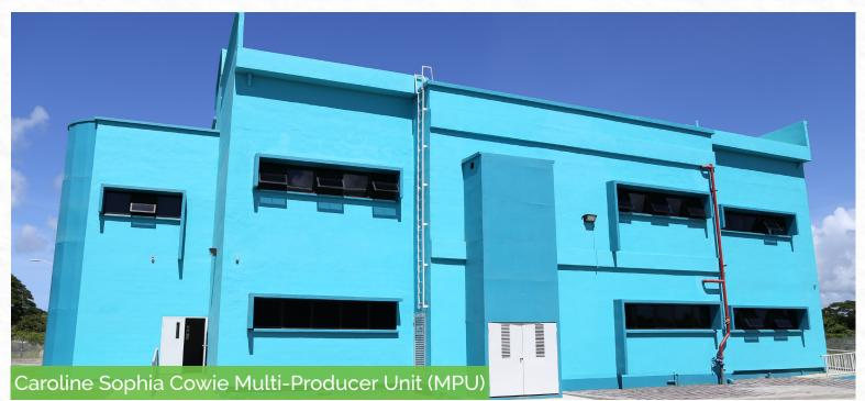
This structural steel-framed building is designed for light manufacturing and agro-processing operations. It comprises two (2) levels, with four (4) units on each level. Each unit ranges from 53.2 m<sup>2</sup> (573 ft<sup>2</sup>) to 130.1 m<sup>2</sup> (1,400 ft<sup>2</sup>) and include common services areas such as a service lift, loading bay, welfare and safety facilities and all supporting infrastructure (electricity, telecommunications and water).
